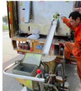
■ The paint heating
